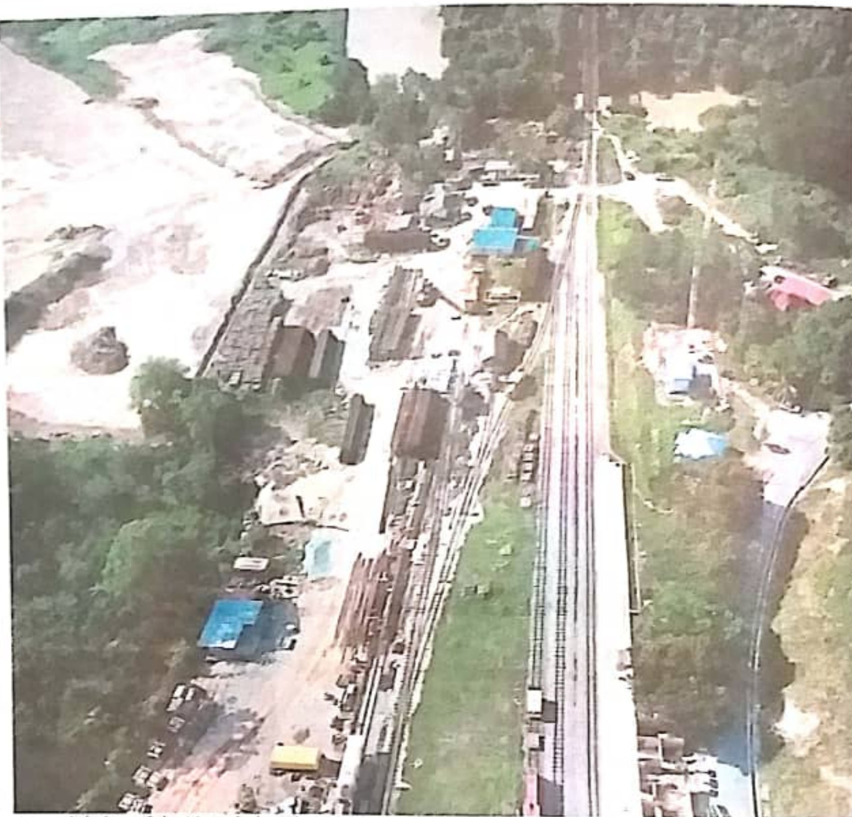
An aerial view of the Mentakab railway station in Pahang. The East Coast Rail Link project is set to be the backbone of the development of Kelantan, Terengganu, Pahang and Negri Sembilan. PIC BY FARIZUL HAFIZ AWANG
