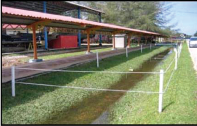
FIGURE 3. Swale drainage at USM (Mustaffa et al. 2016)
