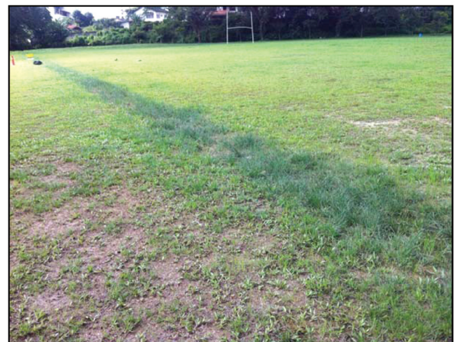
FIGURE 2. Swale drainage at Astaka field
