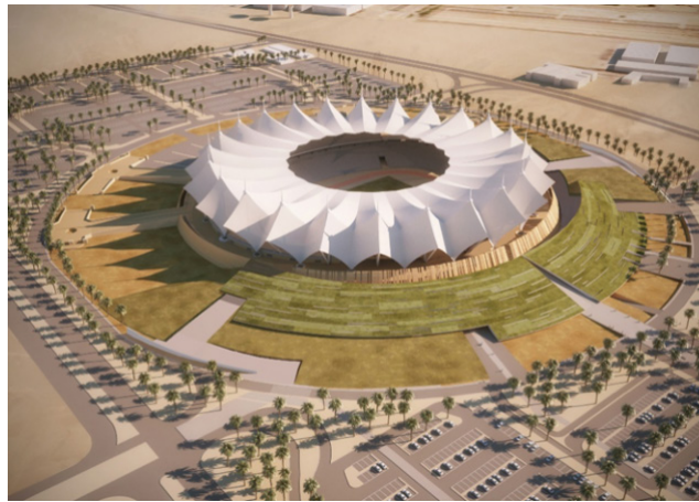
FIGURE 1. Tensioned Fabric Structure
