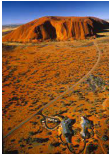
FIGURE 4. Aerial view of Uluru-Kata Tjuta Cultural Centre. Source: Gregory Burgess Architects
