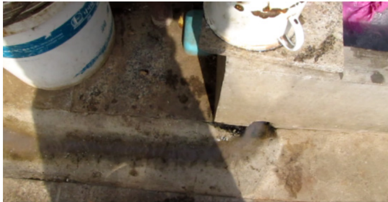
FIGURE 9. Drainage system in the courtyard
