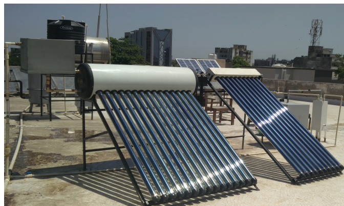
FIGURE 5. ETCs in solar water heater
