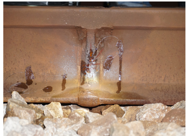
FIGURE 8. The FBG sensors configuration after installation
