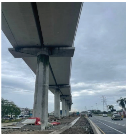
FIGURE 2. Bridge pier structure
