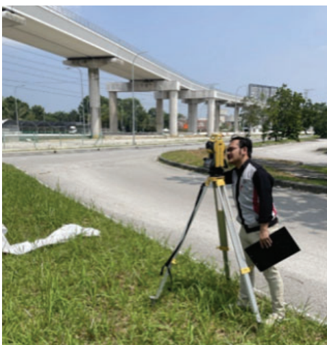
FIGURE 6. Measuring actual data using Total Station
