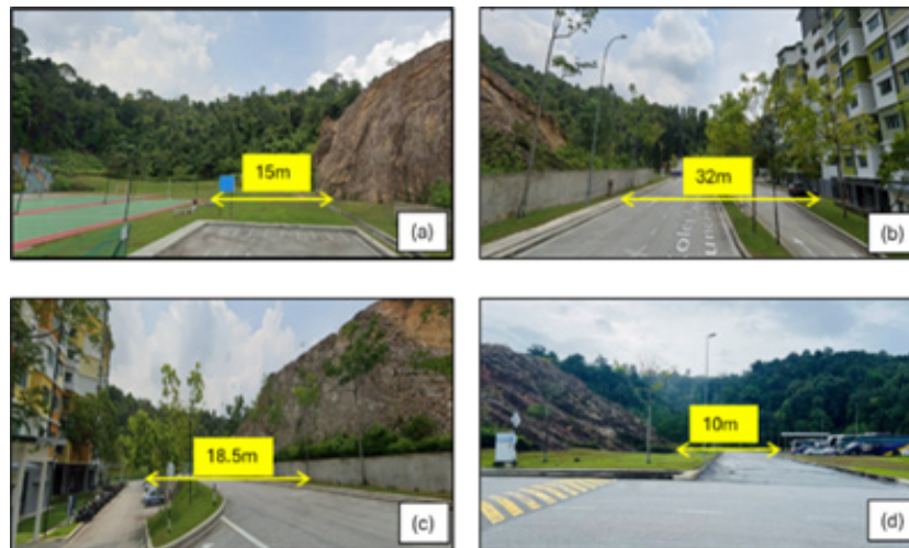
FIGURE 2. Distance of infrastructures to the rock slope (a) Location A; Sport courts; (b) Location B; Kolej Baiduri; (c) Location B; Kolej Zamrud; (d) Location C: Bus depot
