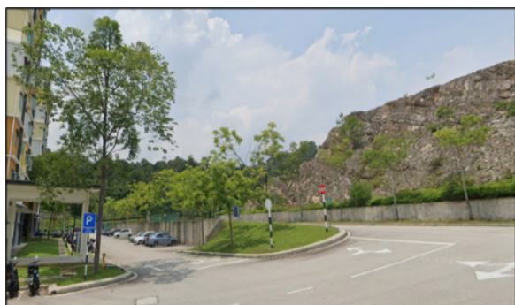
FIGURE 11. Double retaining walls with horizontal drains at Location B
