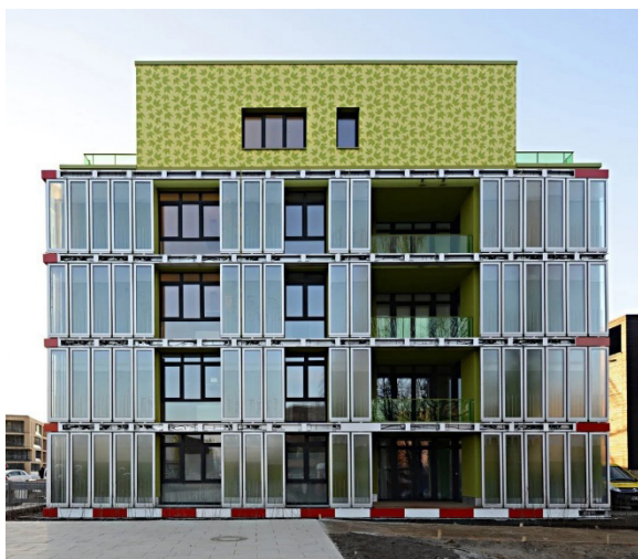
RAJAH 9. Fasad Bioreactor BIQ House
