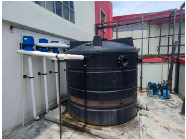
Rainwater Harvesting at Research Complex
