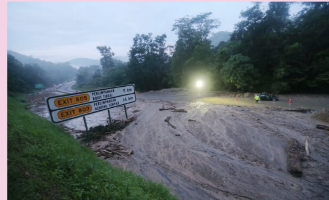
A debris flow occurred at KM52.4 of the Kuala Lumpur-Karak Expressway on 11 November 2015. Photo by NST.
