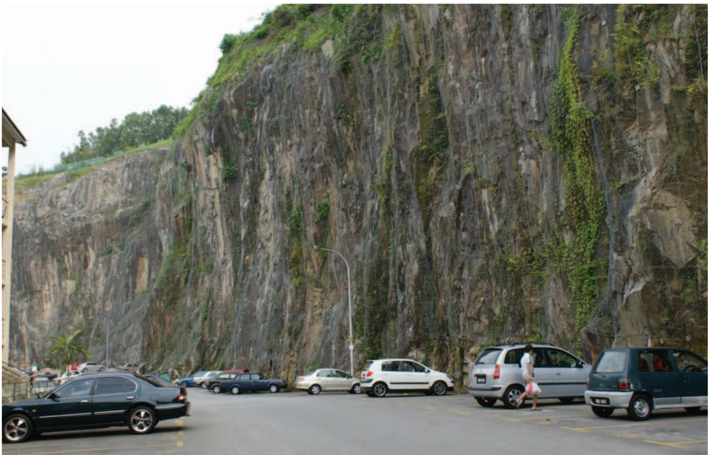
One of the ex-quarry in the outskirts of Kelang Valley, which has been converted into a housing project. There is a high potential for rock fall geohazards at this site
