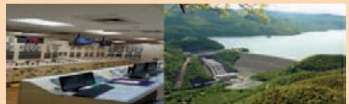
Figure 5: Advanced communication systems for early warning and community engagement by dam authorities play an important role to reduce the vulnerability of downstream populations that are exposed to flooding.
