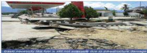
Basic necessity like fuel is still not available due to infrastructure damage.
