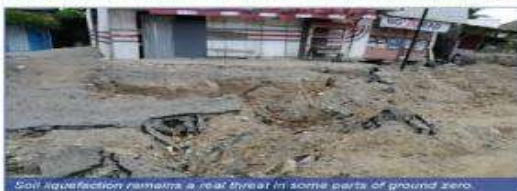
Soil liquefaction remains a real threat in some parts of ground zero.
